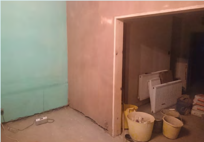
Re-plastering in the living room.
