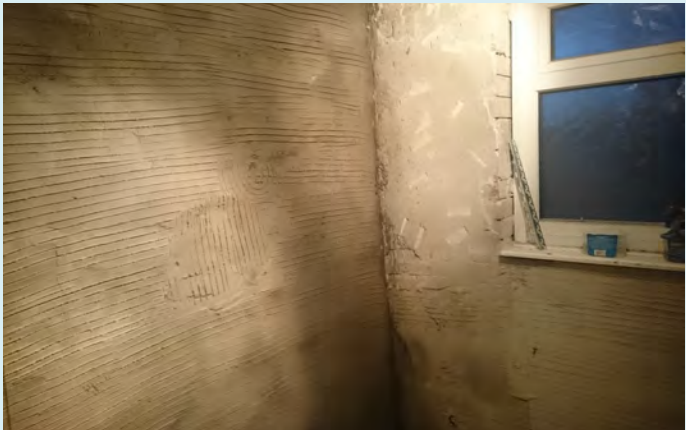
Bathroom tiles were also removed and replaced.
