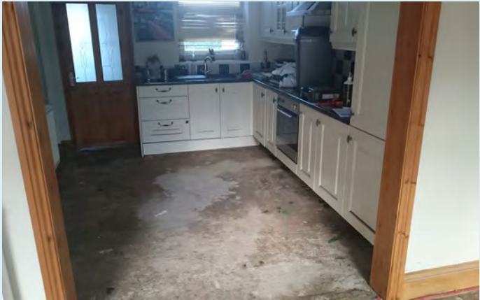
Tiles in the kitchen floor were stripped out and replaced.
