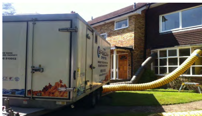
Above: speed drying trailer
