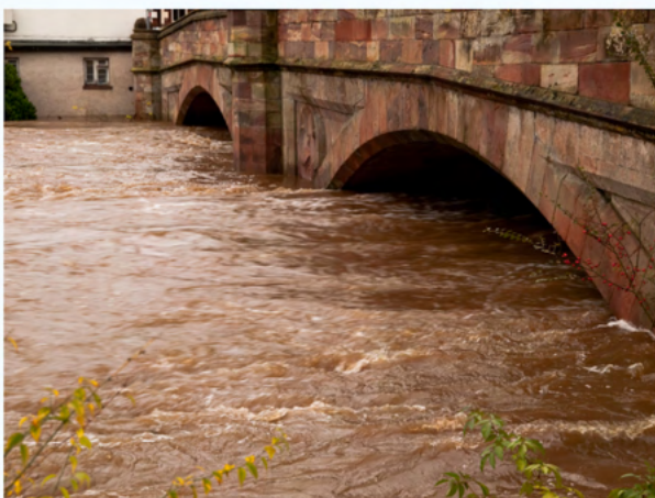
Flooding in Cumbria
